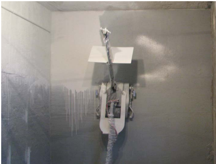
Figure 5. Excessive fixative running down wall during spraying
