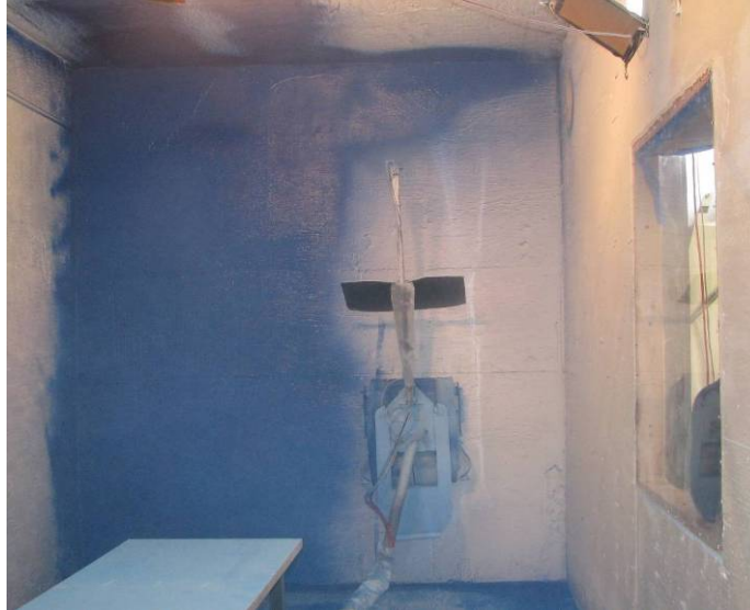
Figure 7. PBS fixative being sprayed on hot cell mockup wall
